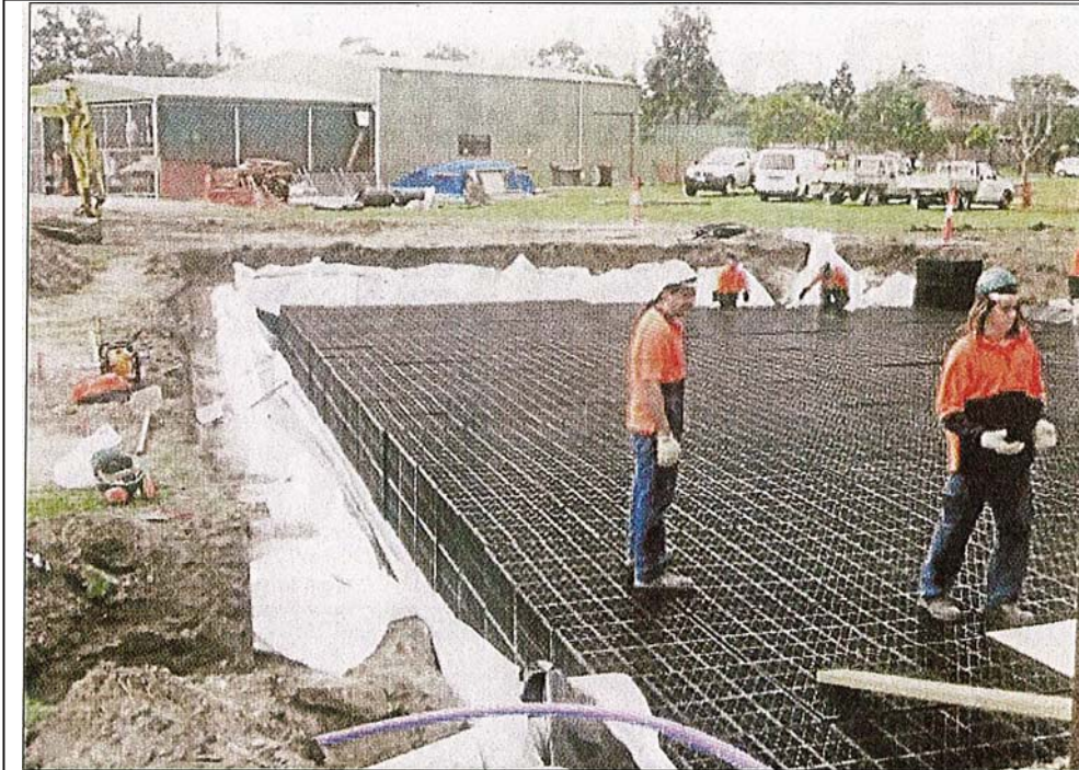
Water wise: Workers install the 180,000-litre tank at Kilbreda College, Mentone.
